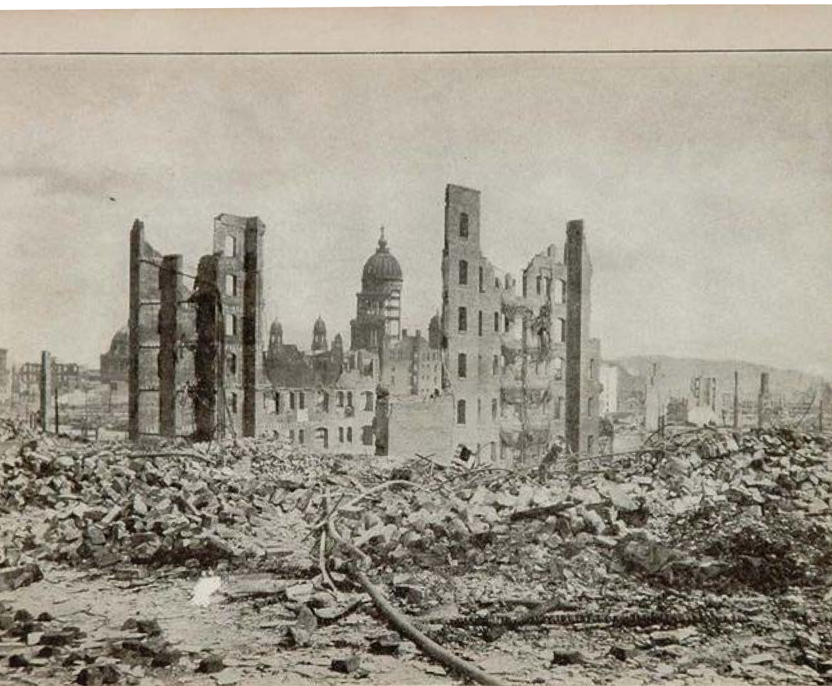
VIEW OF THE RUINS LOOKING TOWARD VAN NESS AVENUE. This photograph, taken at Van Ness Avenue, where a mile of magnificent mansions were blown up to stay the progress of the flames, gives an unparalleled picture of desolation. The ruins of the $7,000,000 City Hall are seen in the distance.
